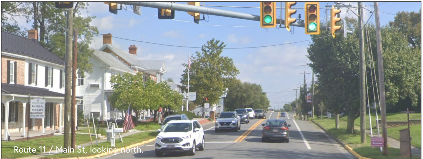
Route 11 / Valley Pike, looking north.
