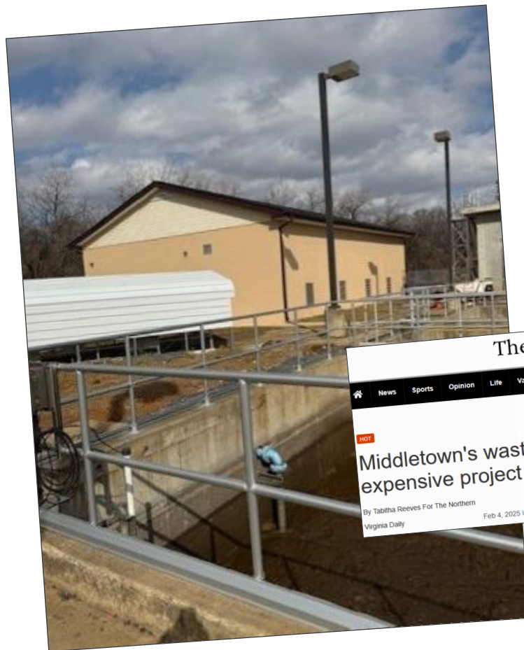
Figure 12. Middletown's Wastewater Plant
